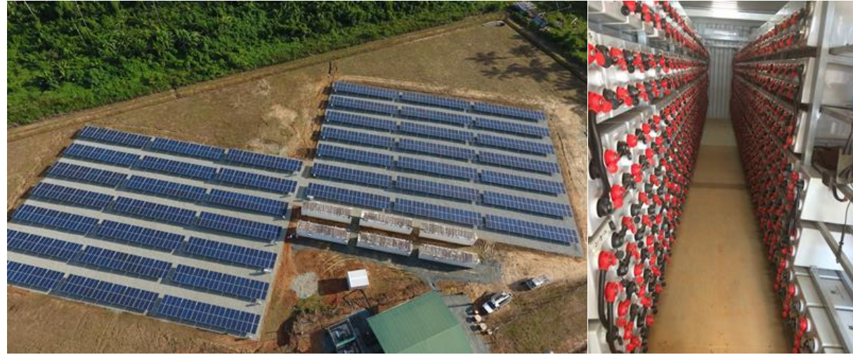
Solar minigrid with battery storage in Suriname.
